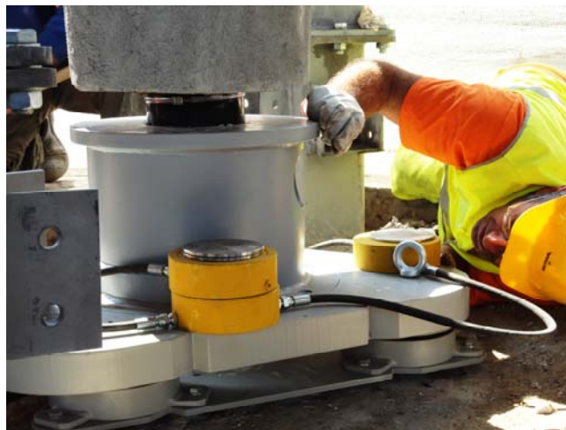
Figure 11. Tripod during the assemblage phases.
