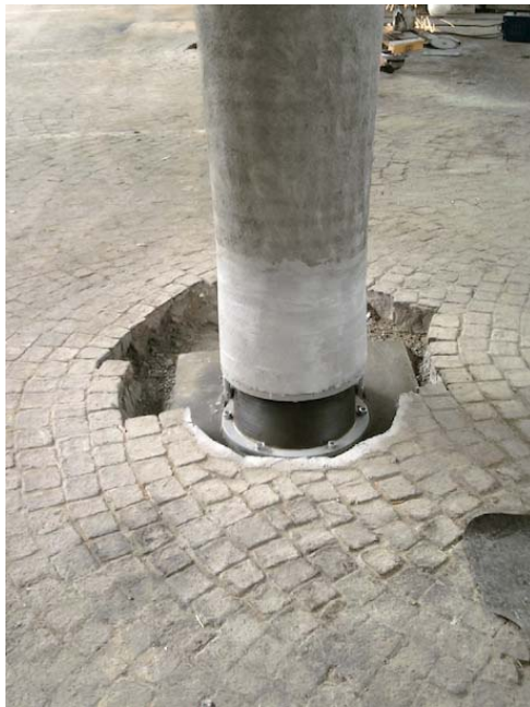
Figure 15. Final configuration of elastomeric isolators.
