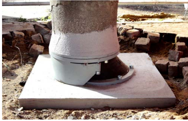
Figure 12. Isolator device with its locking system.
