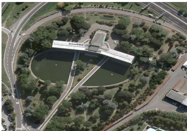
Figure 1. Aerial view of the building.
