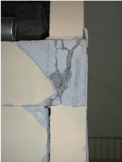
Fig. 1 – Detail of a damaged joint of model No. 3 at the end of the tests in the fixed base condition
