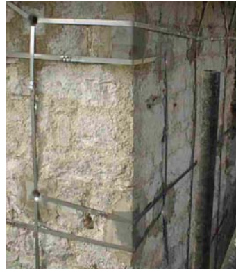
Fig. 11 - Detail of the connection between orthogonal walls.
