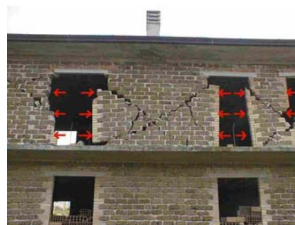
Fig. 2 – Failure mechanism of a new building.
