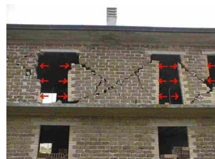
Fig. 2 – Failure mechanism of a new building.
