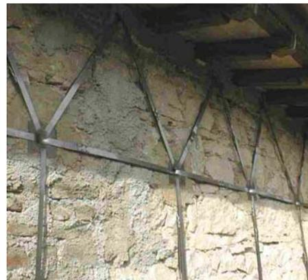
Fig. 9 – CAM arrangement in the facade and link to the top R/C kerb.
