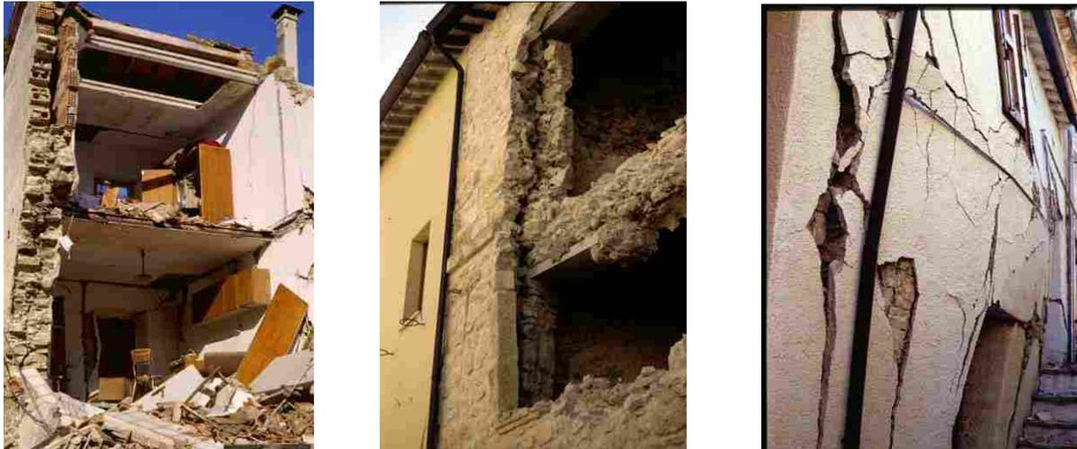
Fig. 1 - Collapse mechanisms of old Italian buildings (Umbria-Marche 1997 Earthquake).
