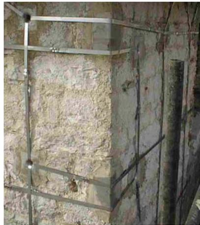
Fig. 11 - Detail of the connection between orthogonal walls.
