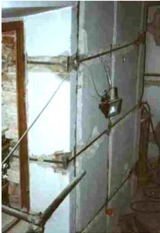
Fig. 10 – CAM arrangement in chase.
