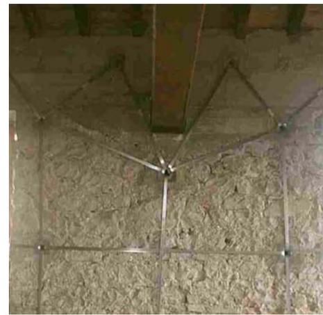
Fig. 12 - Detail of the link to the R/C kerb around a wooden truss.
